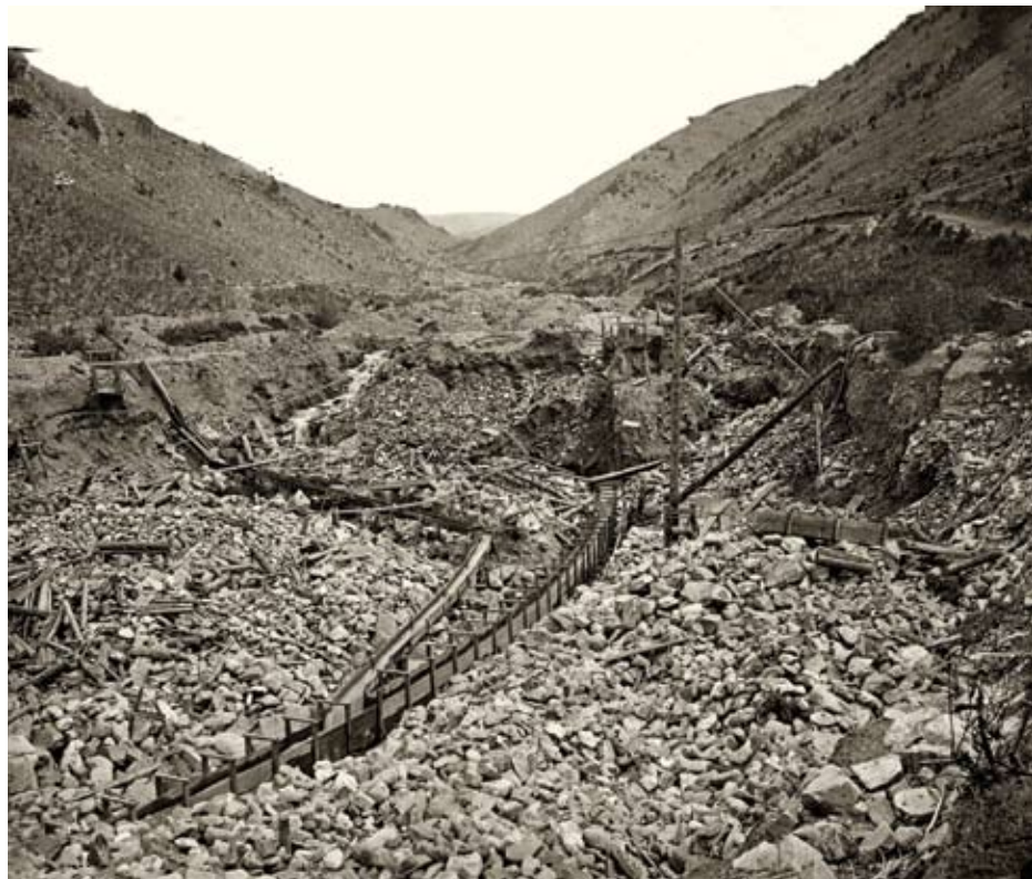
FIGURE 6.3: By the end of the 1860s, Alder Gulch looked like this. Hydraulic mining had eroded the soil down to bare rock, most of the trees were cut down, and wooden flumes (channels) redirected the stream water to the mining operations.
