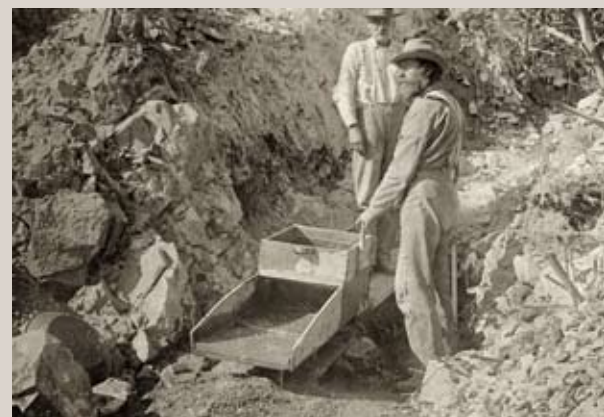
FIGURE 6.22: A rocker was a good two-man method for removing loose gold from dirt and gravel. One man shoveled dirt and gravel while the other worked the rocker.
